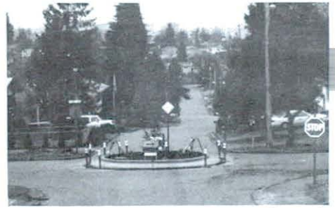
A traffic circle was constructed at the intersection of South 244th Street and 20th Avenue South.
